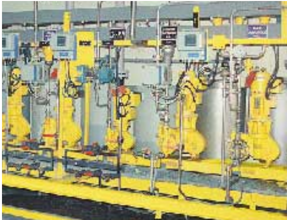
Paper industry : mROY® pumps for bleaching recycled paper.
